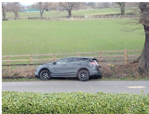
Fig 2: Traffic hazard due to soft verges and deep ditches
