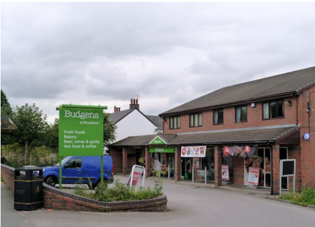
Figure 1: 442 Chester Road, front view of site from Chester Road
